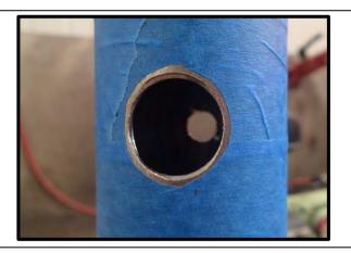
54. Remove all drill/file swarf and then clean and paint with rust preventative paint any exposed/bare metal surfaces left after drilling.
