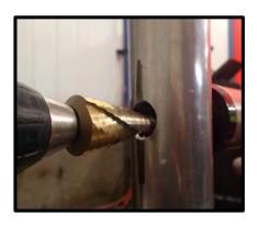
46. Use a stepped drill bit to drill the Ø4mm pilot hole out to Ø24mm.
