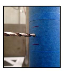
45. At the location of the center mark, use a Ø4mm (or similarly sized) drill bit to drill a pilot hole through the *FRONT* face of the Bull Bar outer frame.
